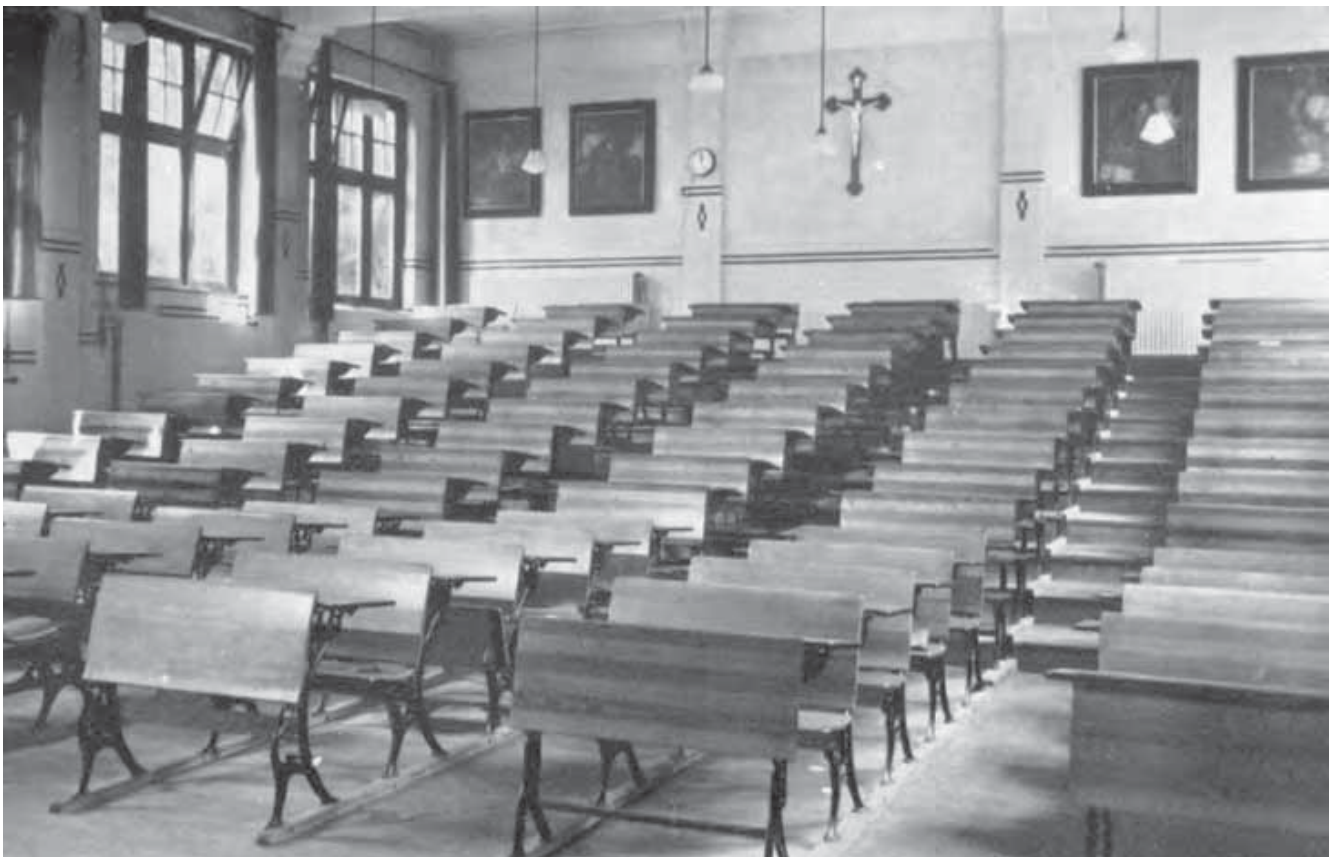
Collegezaal in Warmond. afb. KDC 1a17563
